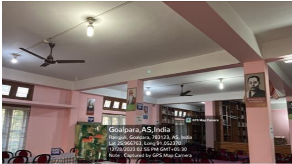
Installation of LED Blubs in classrooms and library
