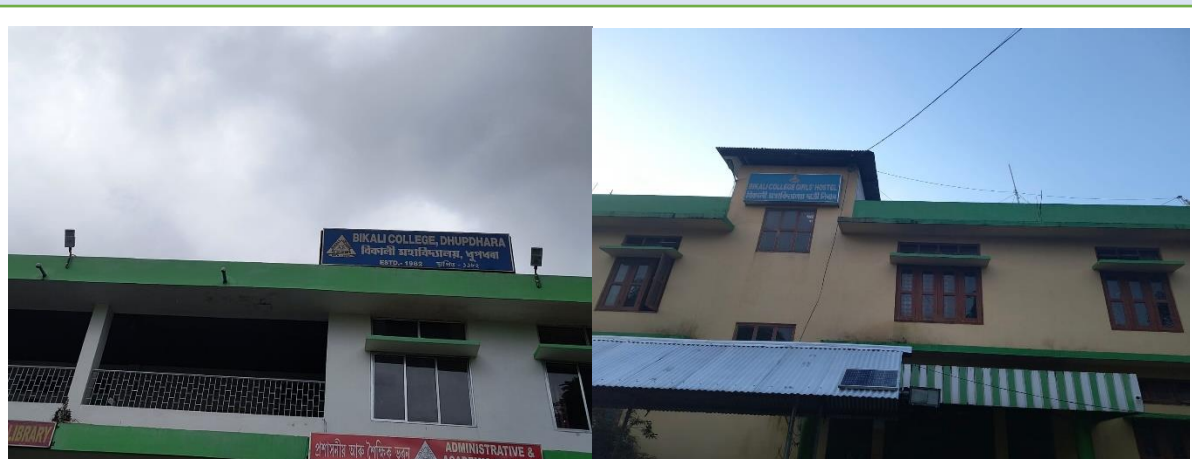
Solar Lights and Panels in different locations
