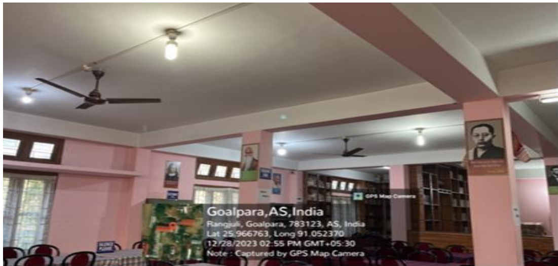
Installation of LED Blubs in classrooms and library
