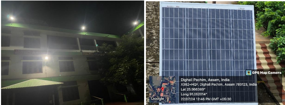
Solar Lights and Panels in different locations
